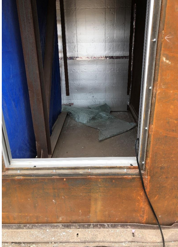
Photo No. 9 Post-test Specimen 16 exterior
