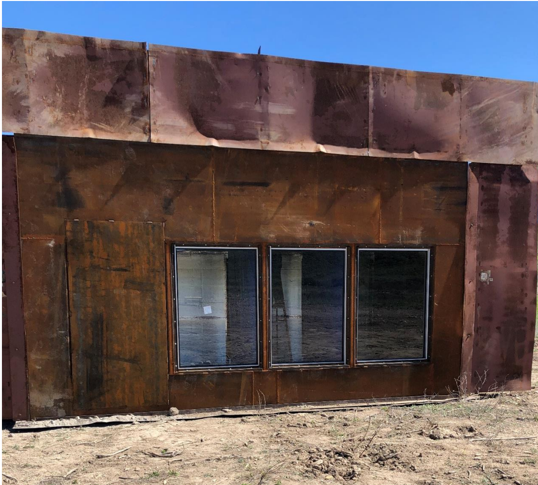
Photo No. 1 Pre-test Specimen 13, 14, 17 exterior
