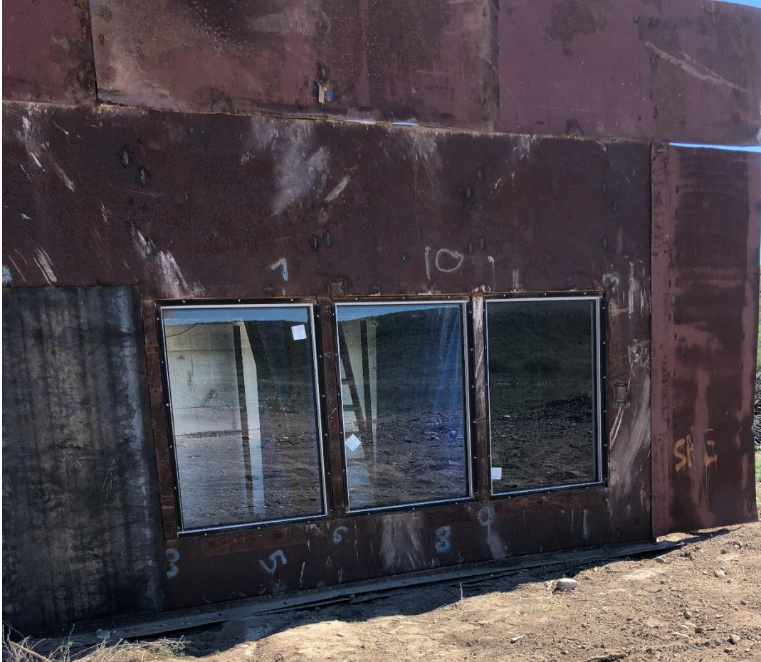
Photo No. 7 Pre-test Specimen 27, 25, 26 exterior
