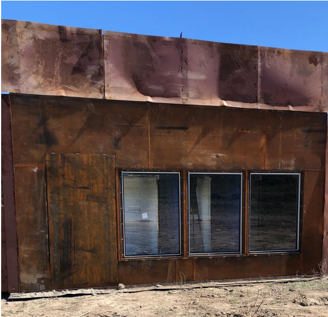
Photo No. 5 Pre-test Specimen 23, 24, 22 exterior
