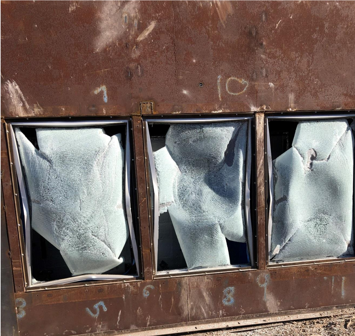
Photo No. 4 Post-test Specimen 20, 19, 21 exterior
