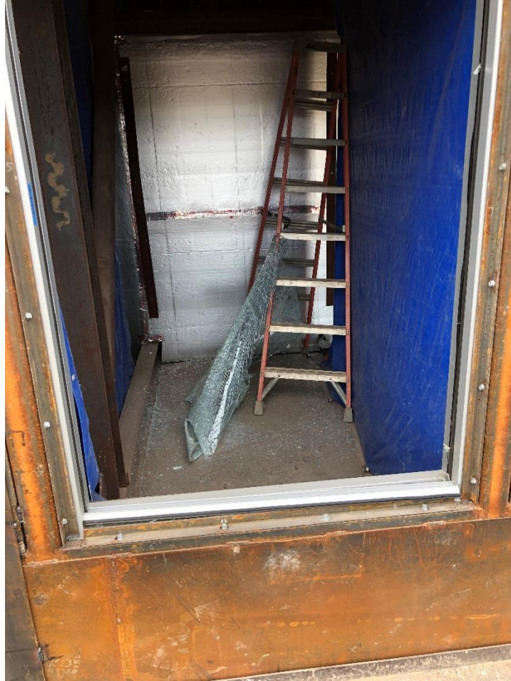
Photo No. 10 Post-test Specimen 18 exterior
