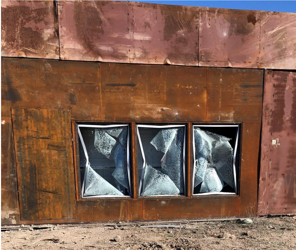
Photo No. 2 Post-test Specimen 13, 14, 17 exterior
